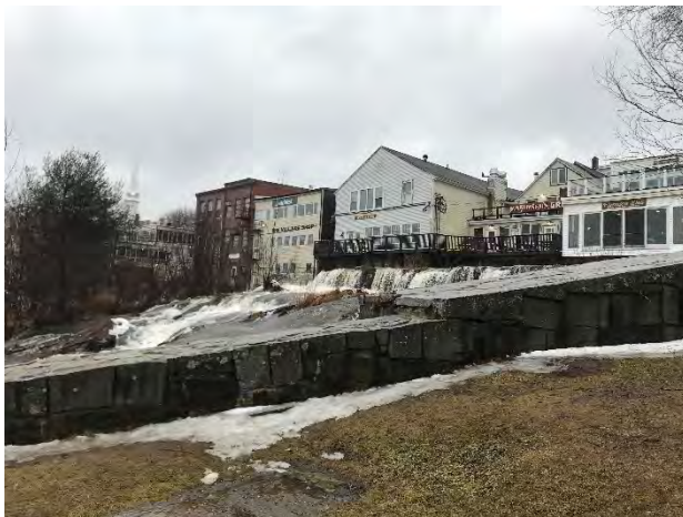
Montgomery Dam Spillway
