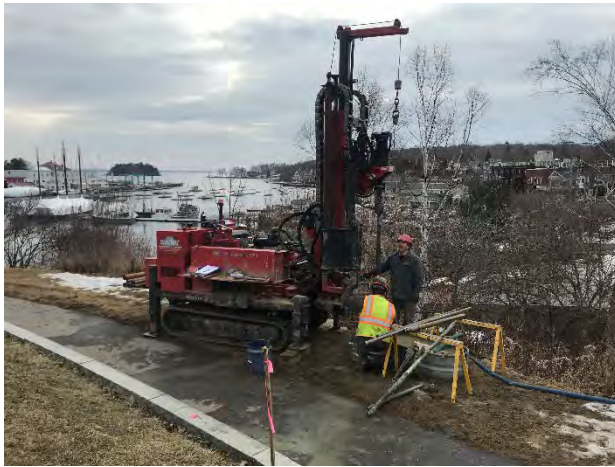
Test Boring B-1 (Rotary Wash)
