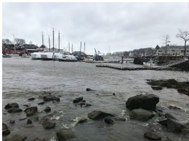
Outlet Below Dam (Harbor)
