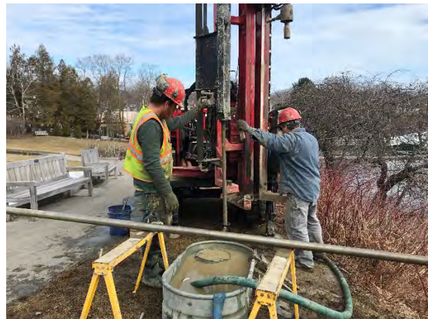
Test Boring B-1 (SPT Sampling)
