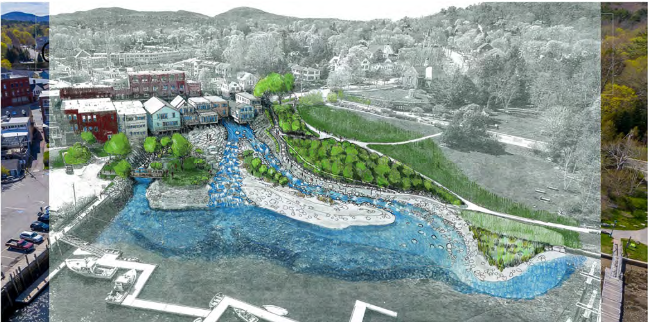
Figure 4. Conceptual rendering of the Montgomery Dam dam removal case with restored channel alignment at high river flow and mean tide level.
